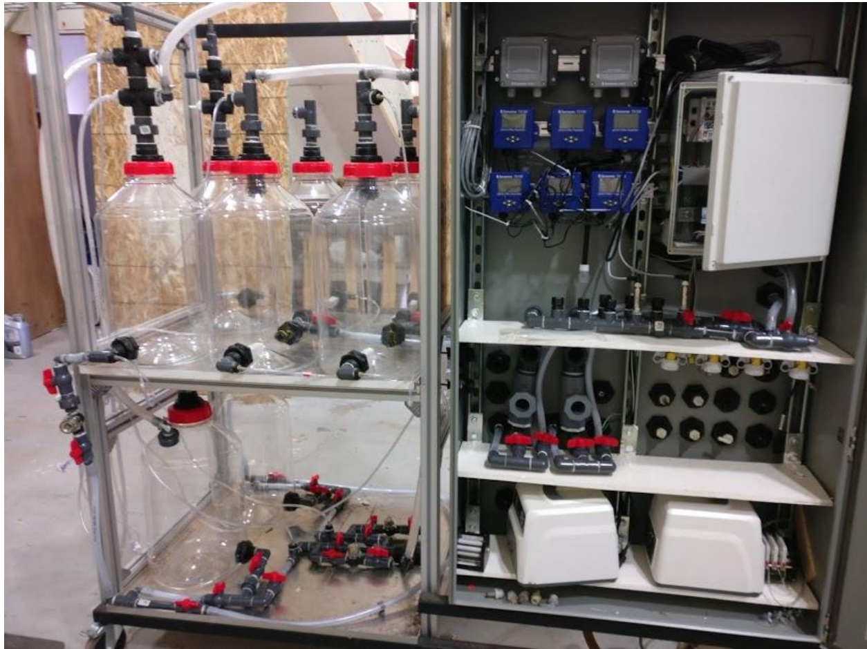
Figure 11 - Photo of electrical cabinet
