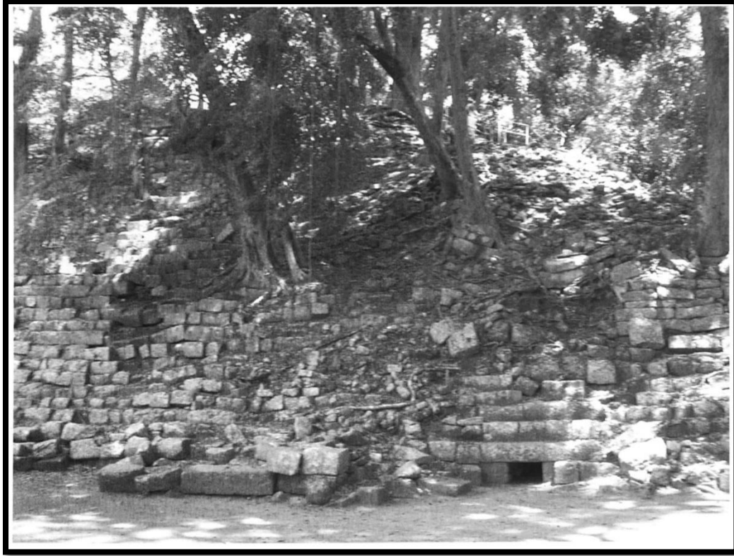
Figure 6.2: Drainage conduit recorded at Copan, Honduras. Adapted from (Davis-Salazar, 2006)
