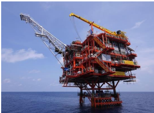
Figure 1-15 Field 3 WPP-A Platform
