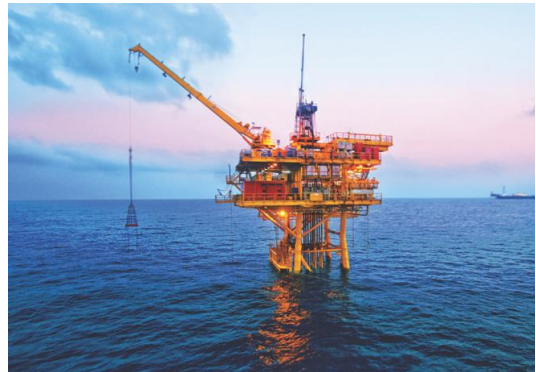
Figure 1-6 Field 1 WHP-A Platform
