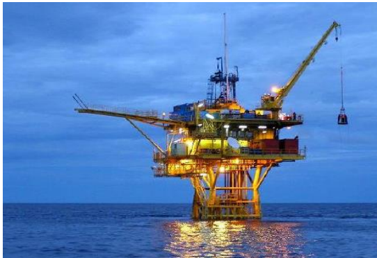
Figure 1-5 Field 1 WPP-C Platform
