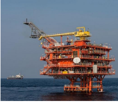
Figure 1-11 Field 2 WPP-A Platform
