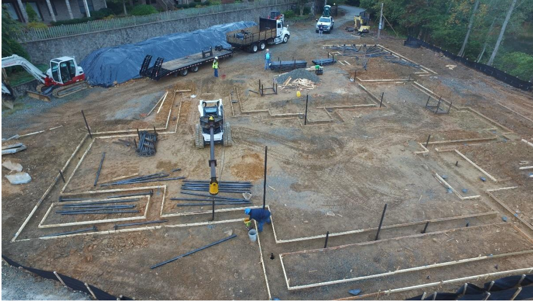
Figure 1.12 Installation of Helical Piles (Courtesy of Cantsink)
