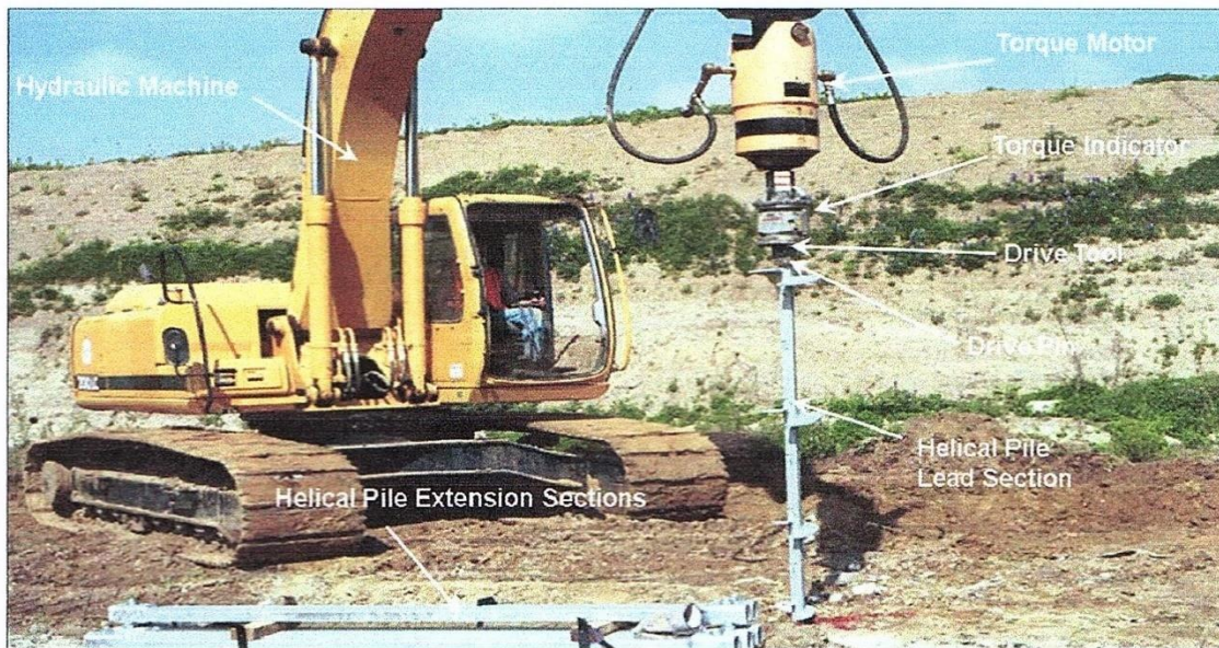
Figure 1.11 Installation equipment terminology (Courtesy of Hubbell Power Systems, Inc)
