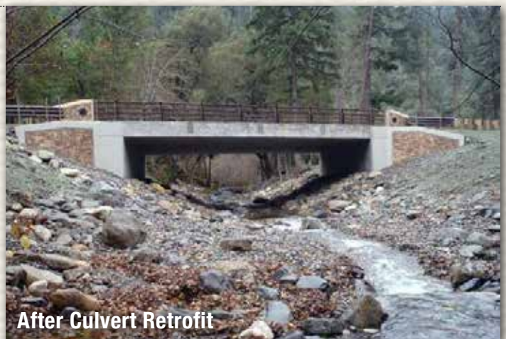
Retrofitting bridge to allow fish passage in Fort Goff Creek, Klamath National Forest, California. Photo courtesy of USFS.
