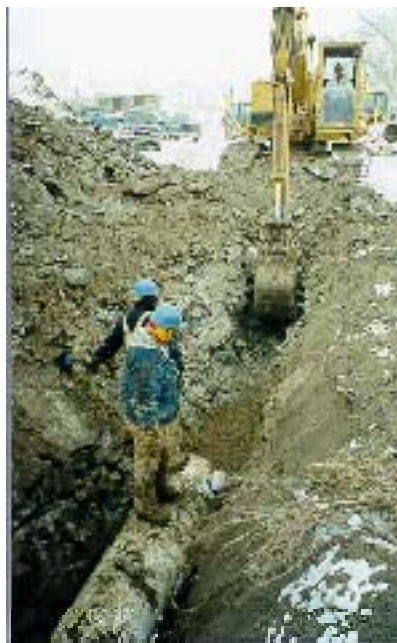
Figure 4. Piping irrigation laterals
