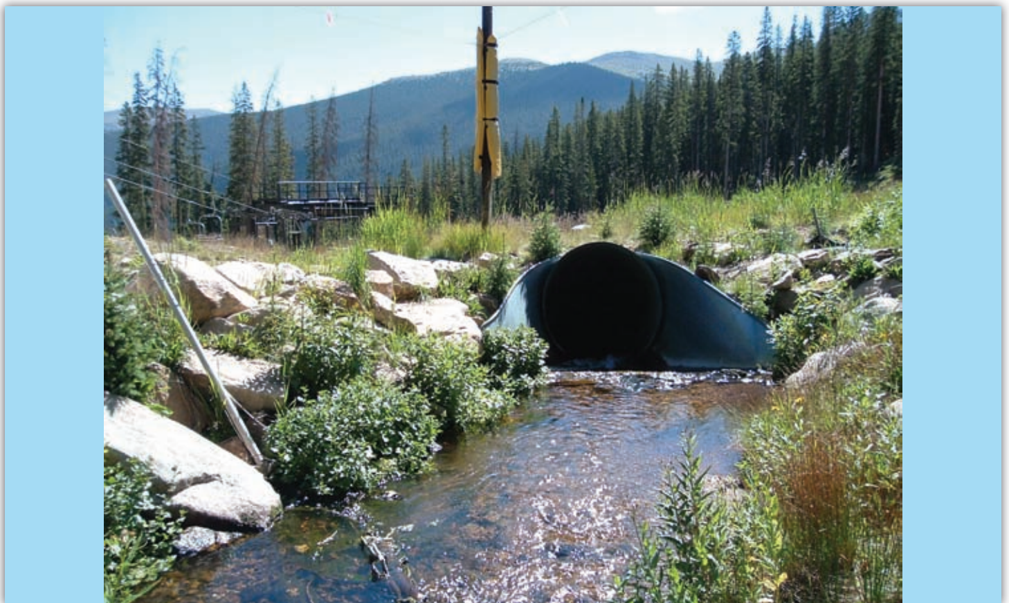
Figure 1. Parsenn Creek enters a culvert under a ski run at Winter Park, Colorado.
