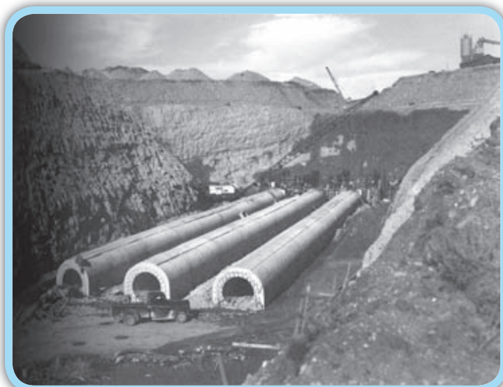
This 1947 photo shows water intakes at the Granby Pumping Plant (Farr Pump Plant).
