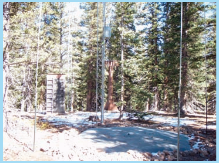
Figure 4. This SNOTEL site was recently installed at Sargents Mesa in the Rio Grande Basin, Colorado.
