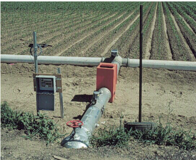
Fig. 1. Surge irrigation system installation
