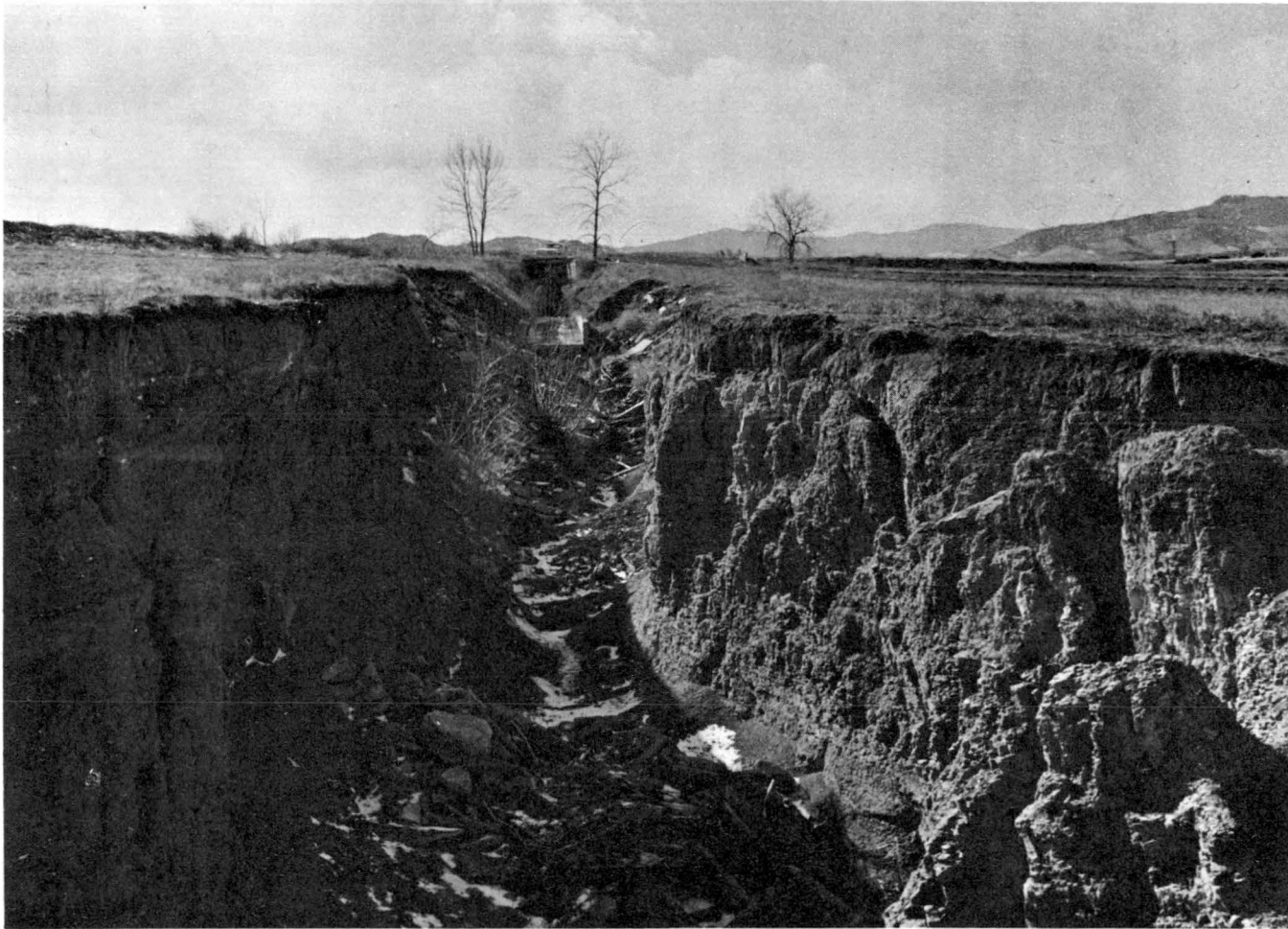
Fig. 8 - Larimer Co. Canal #2 - Warren Lake Channel Erosion
