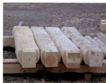
Upper left – front view of panels Left - close-up of scribe-fit joinery Center – end view of panels Above – vertical posts awaiting assembly
