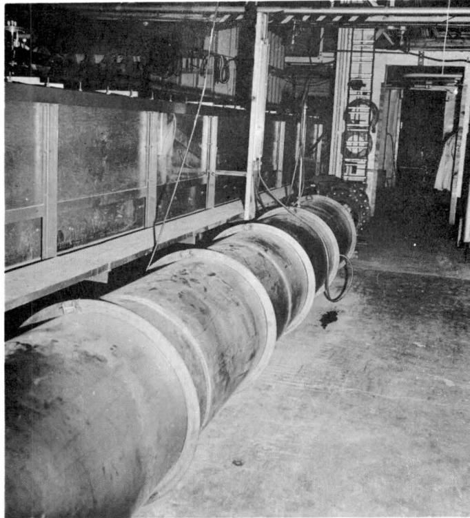
Fig. 3 Meter Installed in 30-Inch Diameter Pipe.
