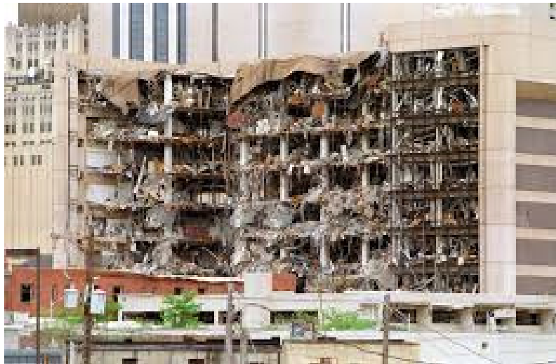
Figure 2.8 Alfred P. Murrah Federal Building in Oklahoma City attack, 1995 (History.com, 2015).
