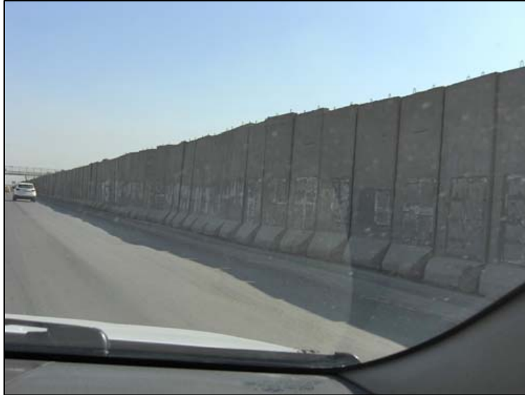
Figure 4.10 Classical blast wall system as used in Iraq (Cathy Breen, 2012).
