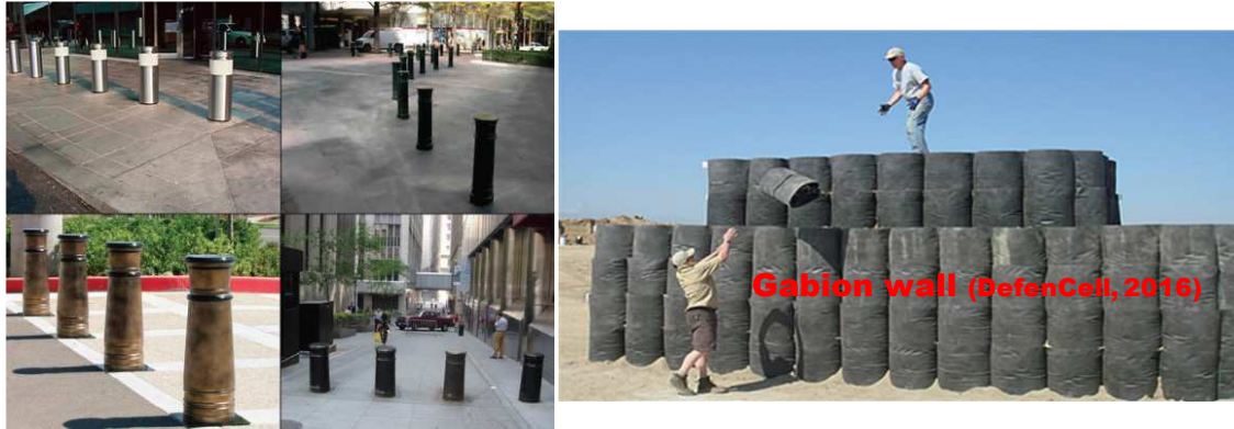
Figure 4.2 Examples of perimeter protection systems.
