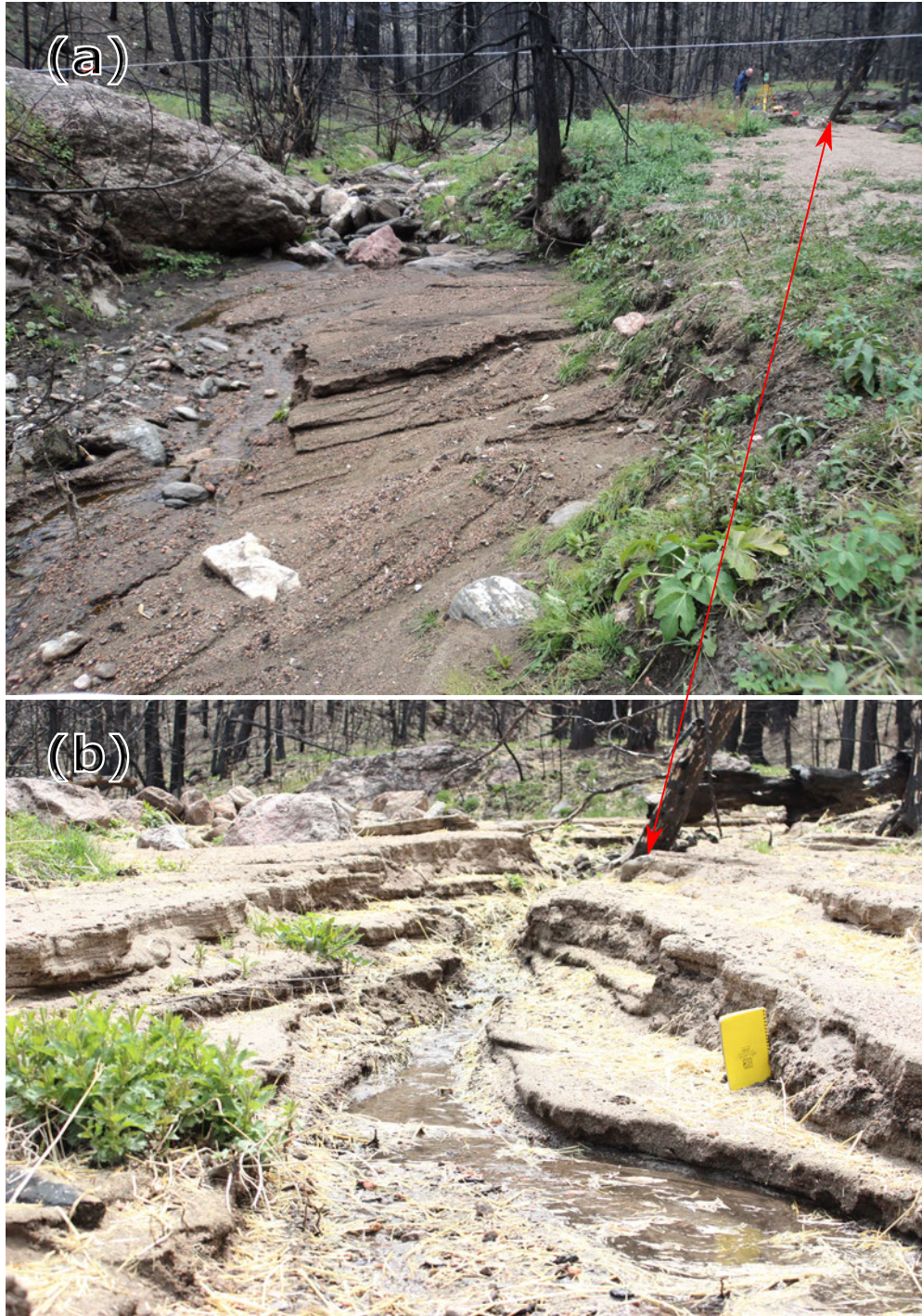
Figure 3.9: (a) Looking upstream at cross section seven (left) and cross section eight (upper right; tributary channel filled with gravel) in Hill Gulch on 22 October 2012 showing deposition following the fire. (b) Looking upstream from near cross section 8 on 12 May 2013 showing the incision during spring snowmelt. The straw mulch in (b) blew into the channel from the adjacent hillside where it had been applied to reduce erosion.
