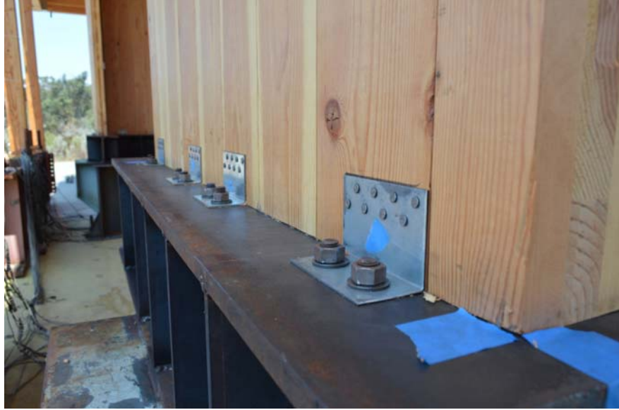
Figure 4.82: Test Configuration 3, Loma Prieta MCE, Perpendicular walls
