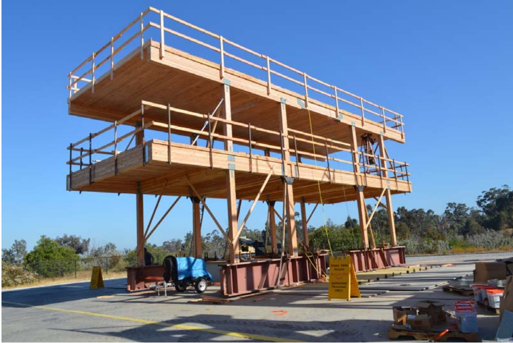
Figure 4.54: Specimen under construction, only gravity frame is seen in the photo
