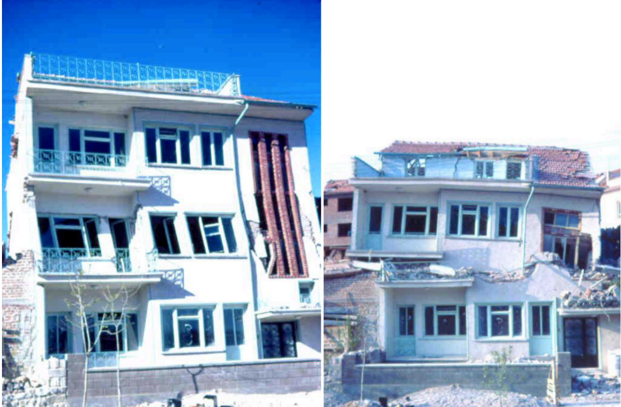
Figure 2-1. Reinforced concrete structure before and after the aftershock event from (Abdelnaby 2012)
