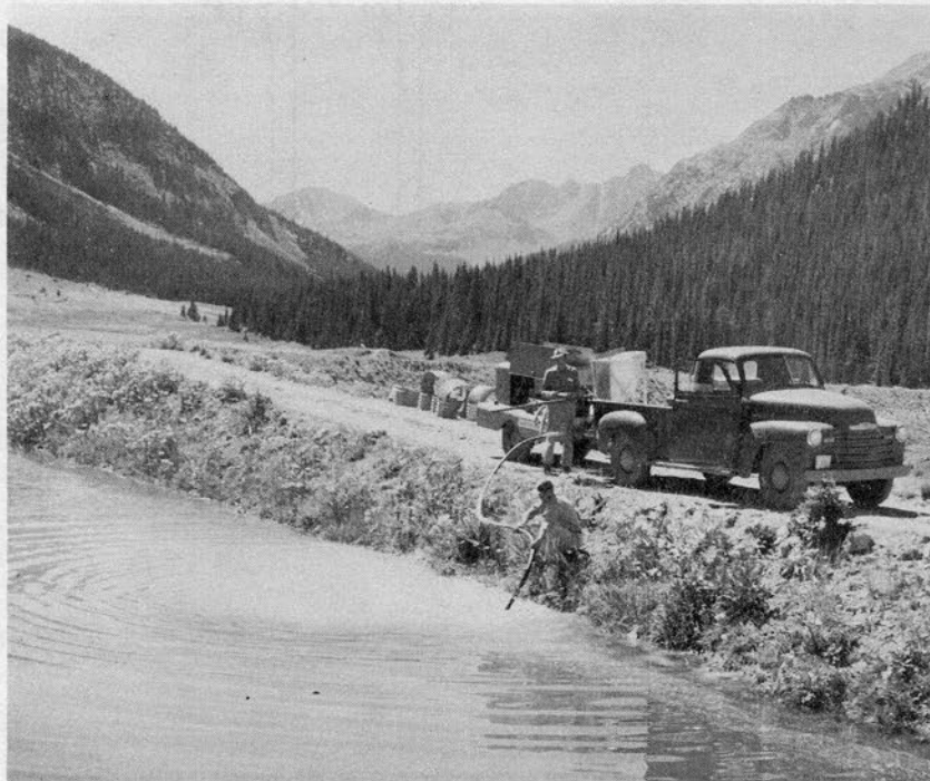
Fig. 44 Bentonite air-jetting with discharge under water
