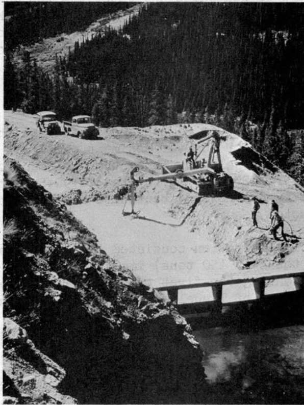
Fig. 35 Mixing bentonite with back-hoe at head end of the Connection Canal
