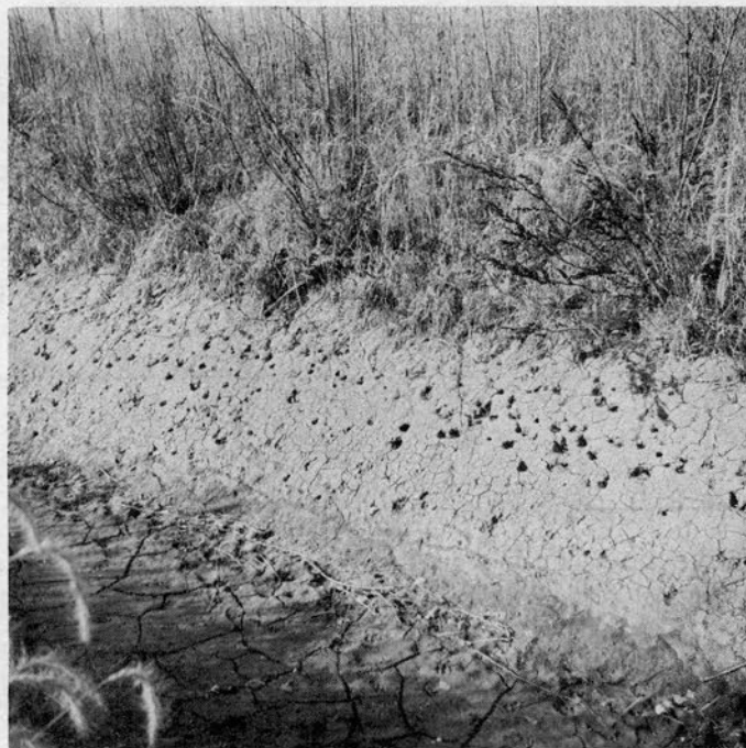
Fig. 5 Crayfish burrows in Lateral 19.3 near Mi. 4.2
