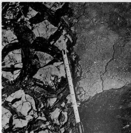
Fig. 31 Drying cracks in bentonite sediment layer in the lateral 1 trial
