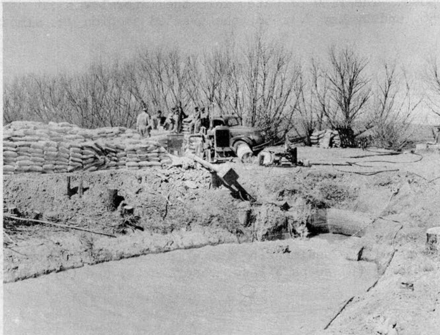
Fig. 29 Bentonite mixing operation for the Lateral 1 trial
