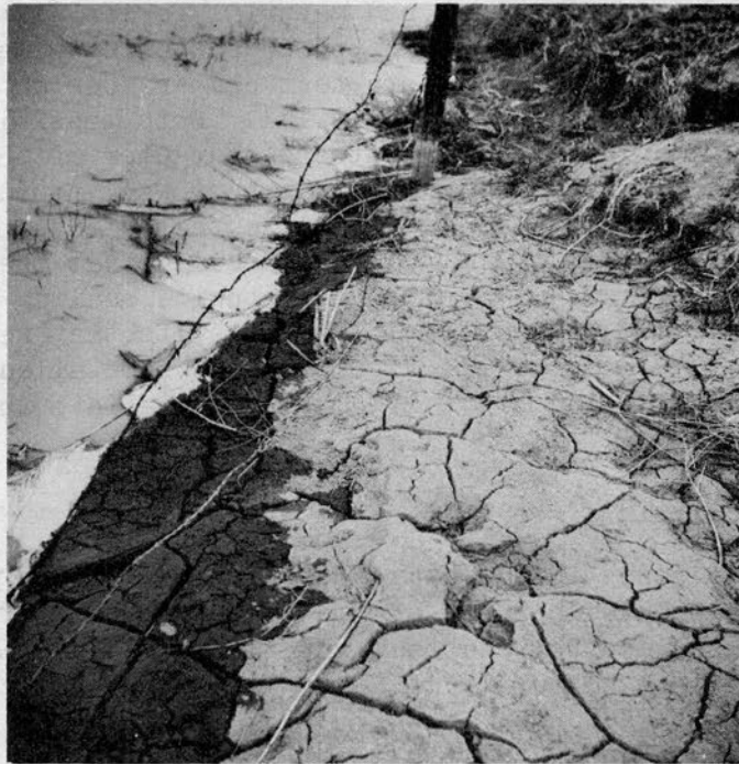
Fig. 4 Drying cracks in loessial material
