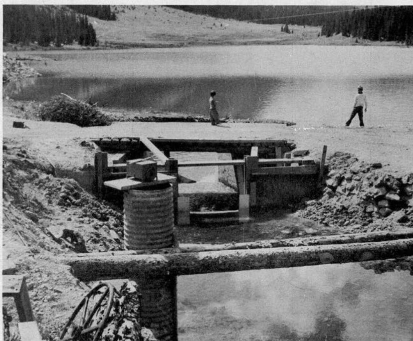
Fig. 38 View of temporary weir installed at lower end of the Connection Canal
