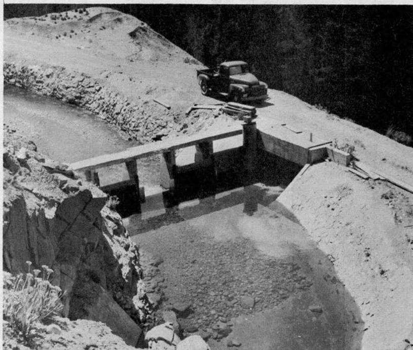
Fig. 37 View of temporary weir installed at upper end of the Connection Canal
