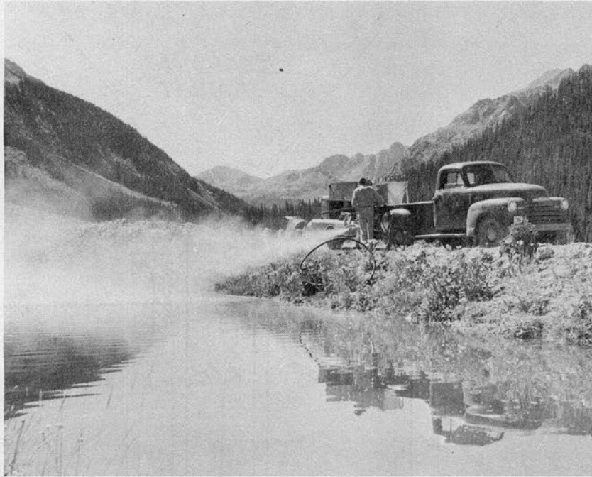
Fig. 43 Bentonite air-jetting with discharge into the air
