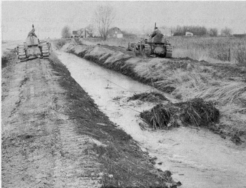
Fig. 8 Harrowing in Pond No. 4 in Lateral 19.3 trial
