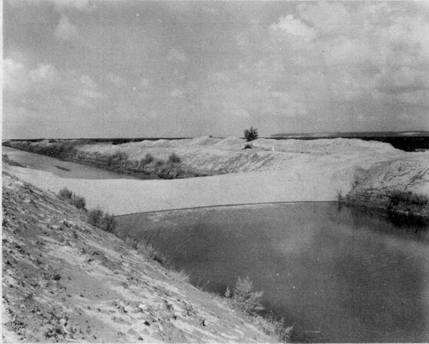
Fig. 23 View looking downstream at the earth dam at Sta. 730+00 during SS-13 ponding
