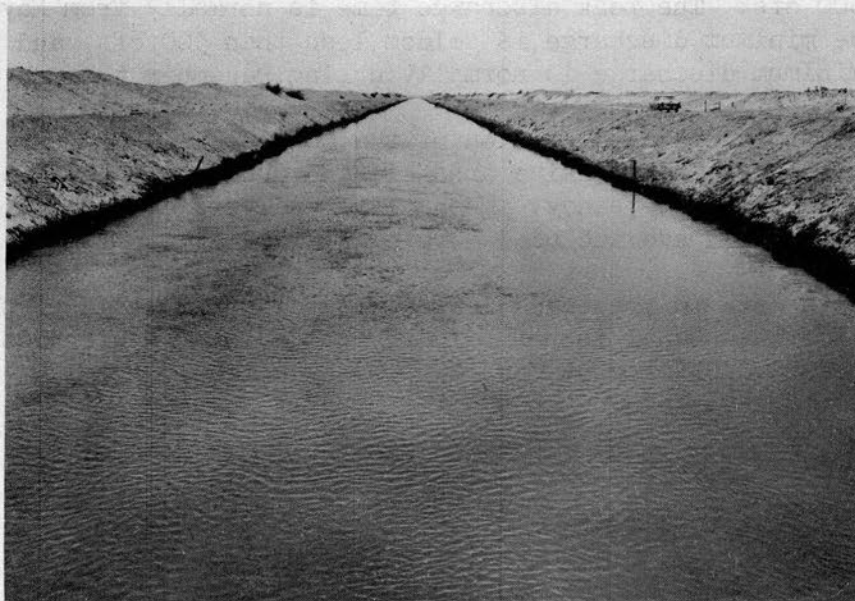
Fig. 12 View of the Coachella site upstream from canal bridge at Sta. 713+10
