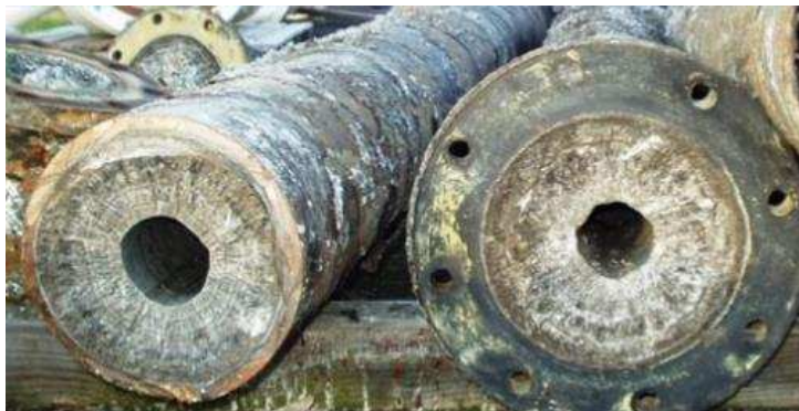
Figure 7- Accumulated struvite formation in WWT pipes (Suszyński, 2016)
