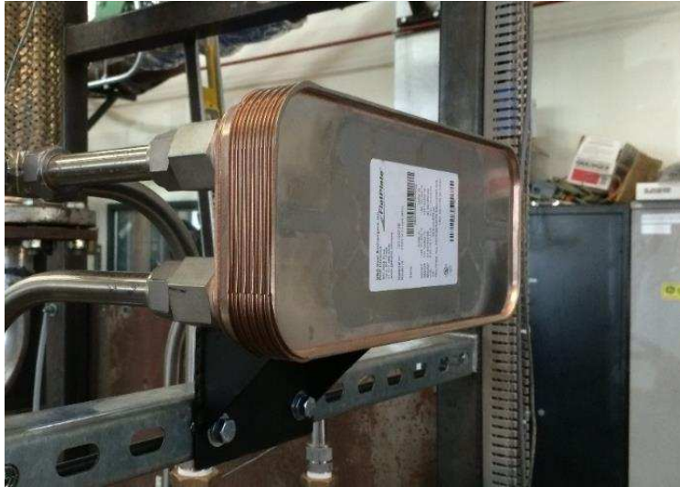
Figure 3-11. Brazed flat plate heat exchanger used to reject heat from primary coolant to secondary coolant.
