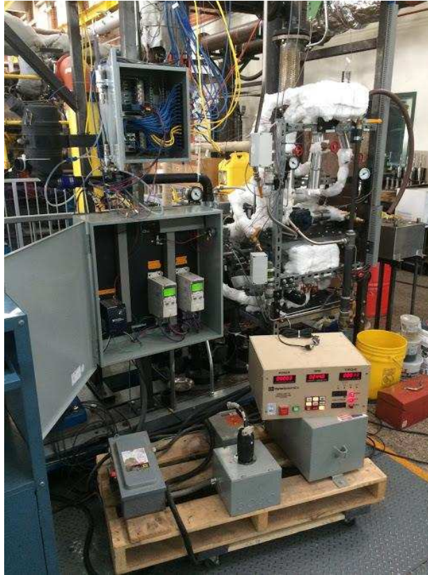
Figure 3-8. Completed test facility including dynamometer controller in the bottom of the image.
