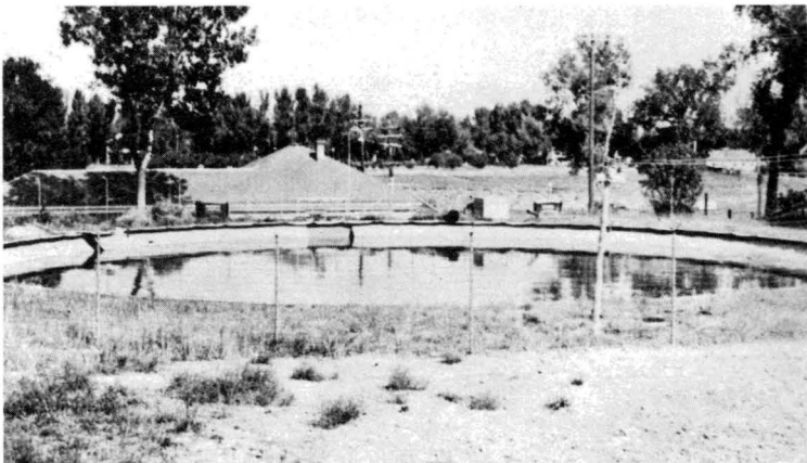
Reservoir and evaporation tank
