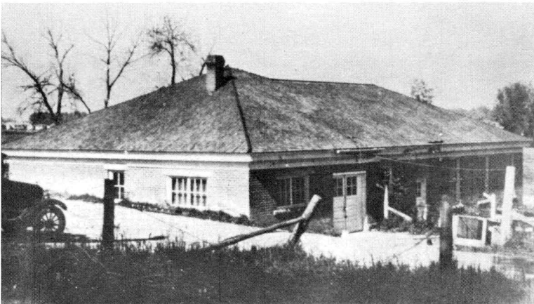
First Hydraulics Laboratory Building
