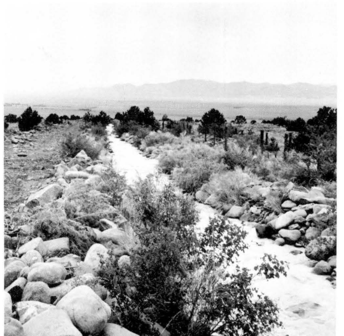
Figure 3.—The milky slurry is carried downstream, sealing where water is lost by seepage.
