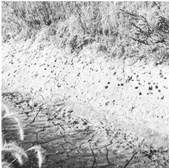
Figure 13.—Crayfish burrowing and deep cracking upon drying is harmful to clay sealing.
