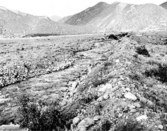
Figure 5.—Channel erosion can produce a short life of sealing.
