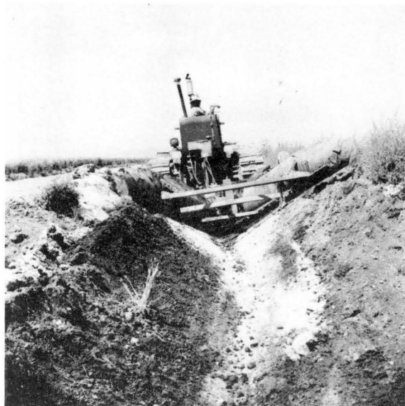
Figure 12.—The clay may be placed in the canal in dams and then mixed into the soil with a V-ditcher.
