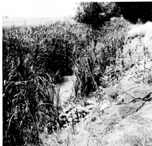
Figure 9.—Adequate channel cleaning, prior to the clay sealing treatment, is a problem in some instances.
