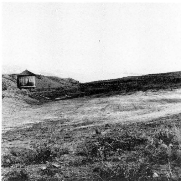
Figure 10.—Mixed layer membrane. Clay is spread over the pond bottom and then harrowed into the soil.
