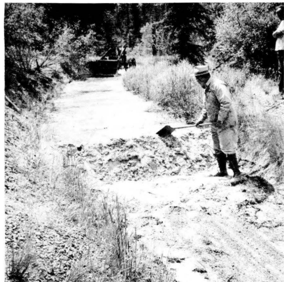
Figure 8.—The slurry is ponded behind the next dam downstream and the breakout process repeated.
