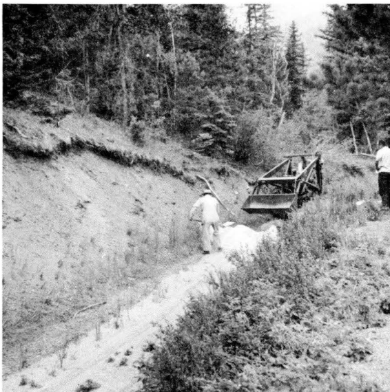
Figure 6.—Dams of clay are spaced along the canal reach being sealed.
