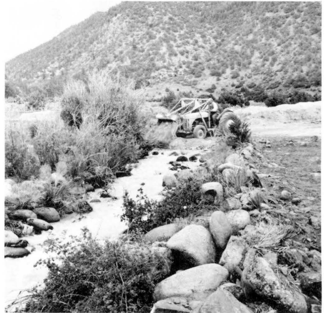
Figure 2.—Clay is washed into the water at the upstream end of the section to be sealed.
