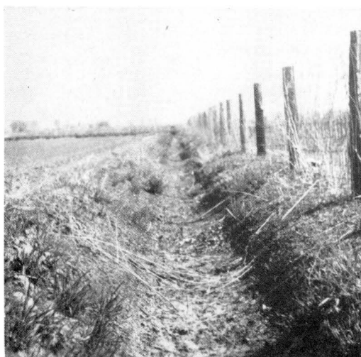
Figure 15—Farm lateral, College East Farm, Fort Collins, Colorado, before being lined.
