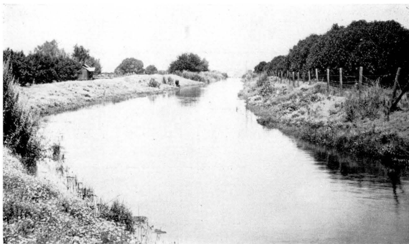
Figure 22.—East Branch Alta canal showing section under test for seepage losses.
