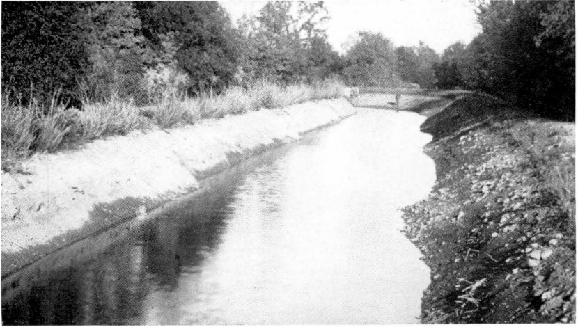
Figure 29.—Anderson-Cottonwood canal, Redding, California, showing canal section and type of soil.
