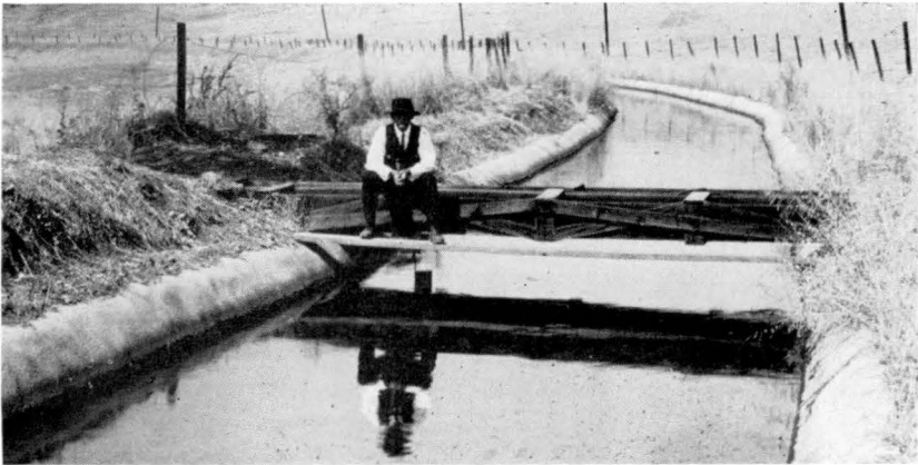
Figure 20.—Lindsay-Strathmore Lowline canal with gunite lining when tested for seepage losses.
