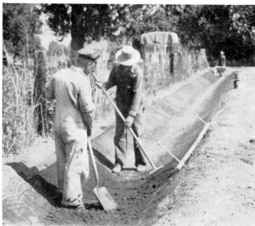
Figure 18.—Oil lining of farm lateral, College East Farm, Fort Collins, Colorado.
