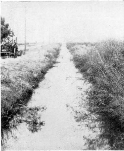
Figure 11.—Pool in Lateral No. 2 North, East Contra Costa Irrigation District, Brentwood, California. Condition of banks is also shown.
