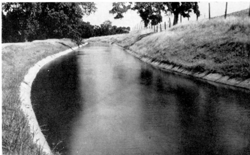
Figure 32.—Concrete-lined Highline Canal, Orland Project, Orland, California.
