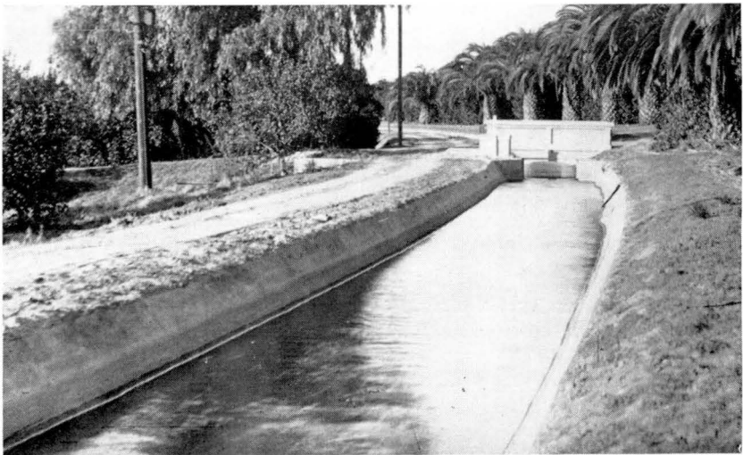
Figure 26.—Concrete lining of Gage Canal at Riverside, California.
