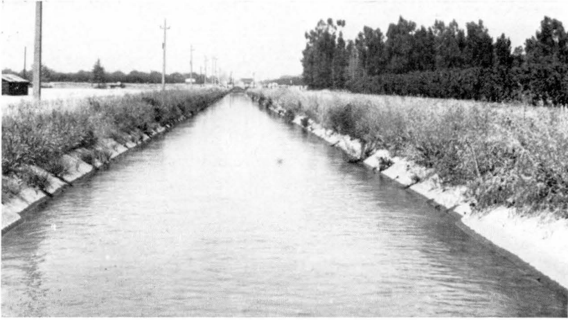
Figure 9.—Portion of pool in East Contra Costa main canal basin, Brentwood, California.
