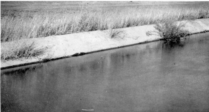
Figure 10.—Cracks in concrete lining of East Contra Costa main canal basin, Brentwood, California.
