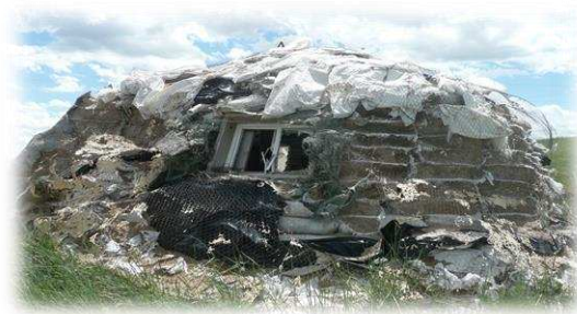
Picture 11- Example of failed project
