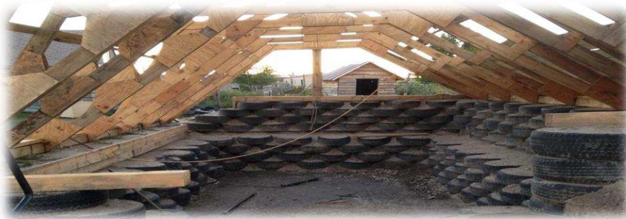
Picture 6- "Walipini" ground greenhouse construction
