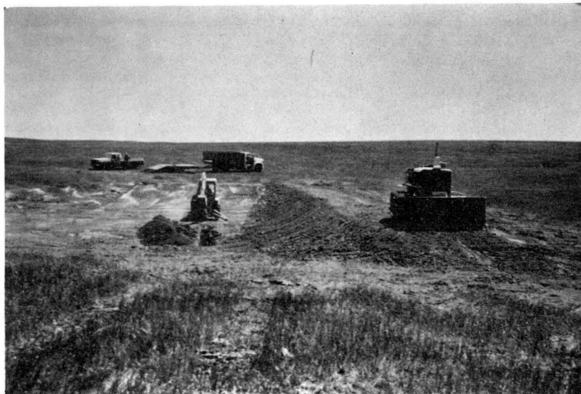
Figure 20. Construction of Earthen Dike (Pine Ridge Site) (Corey and Smith, 1970)
