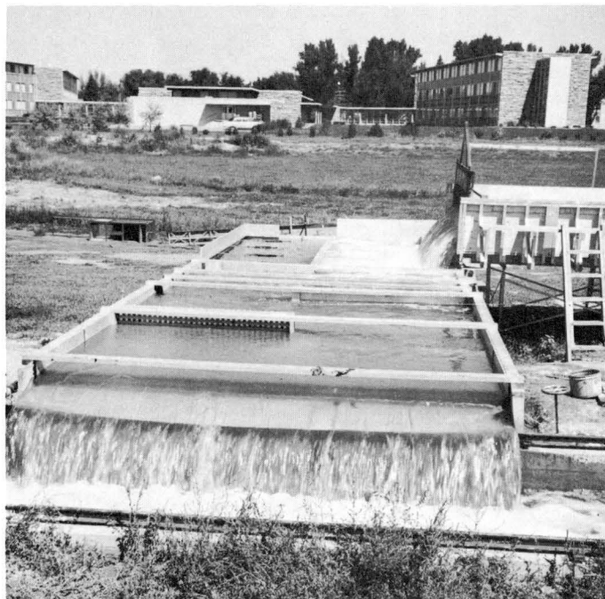
Fig. 10. Tail box. Made purposely large to settle bed material.
