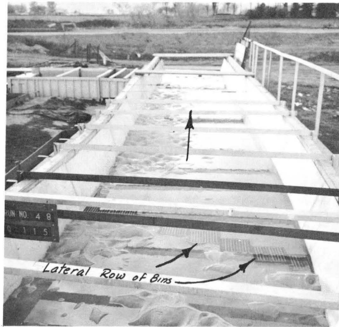
Fig. 29. Lateral ejector bins in canal curve.
