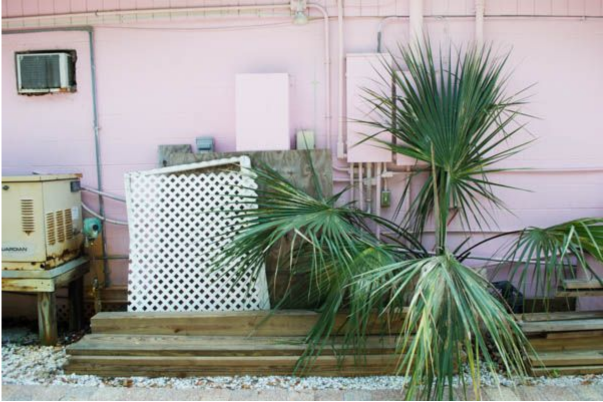
Figure 1: Back of the Shack
