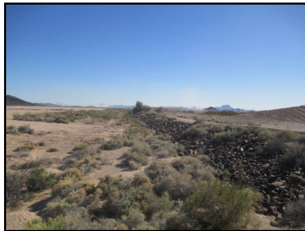
Figure 1: Desert Valley Plain of Watershed near the Levee
