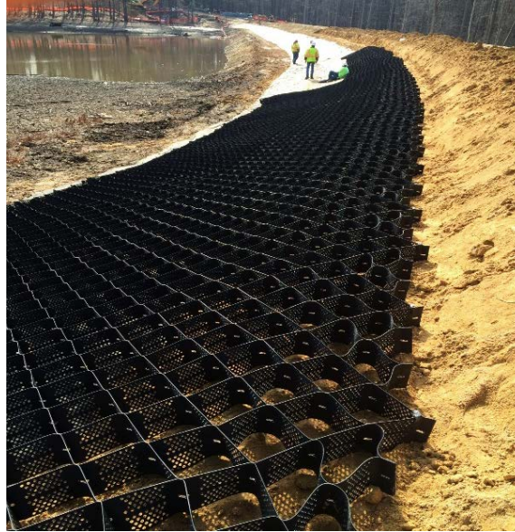
Figure 7. Typical Geoweb System
