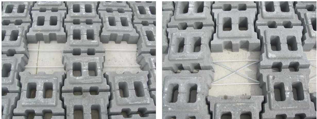
Figure 6. Lacing Detail
