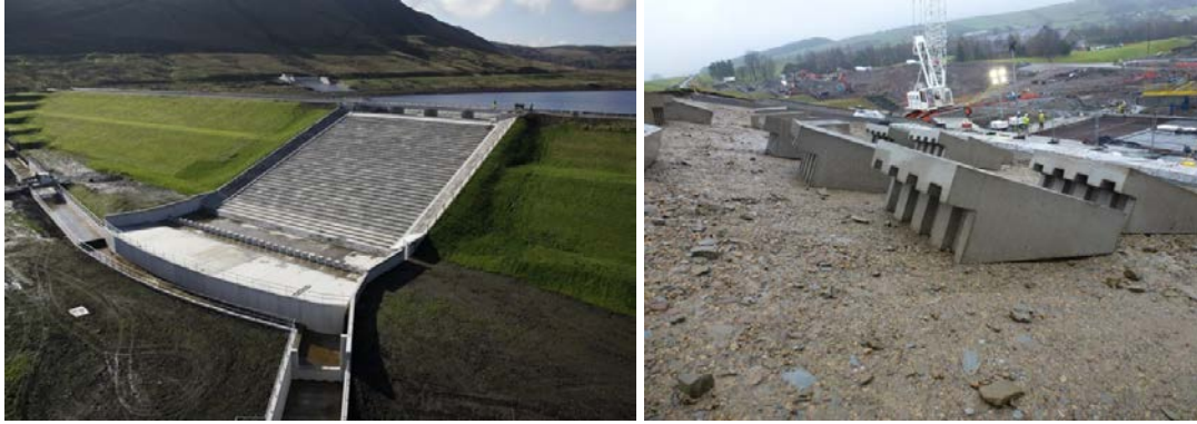
Figure 20. Odgen Dam. Left, downstream view. Right, WSBs before the installation (courtesy of P. Thurlwell, from Pascoe, P&S Consulting Engineers, Ltd.)
