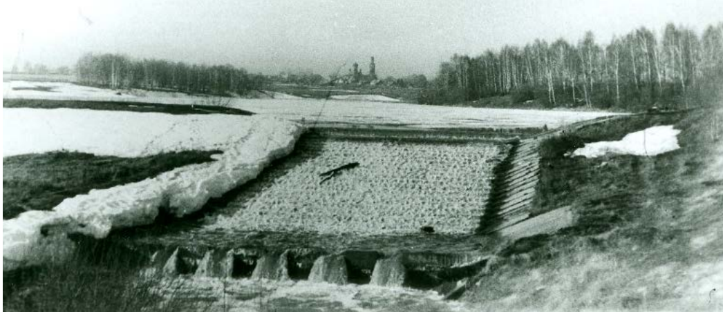
Figure 18. Downstream view of Klinbeldin Dam (courtesy of R. Baker)
