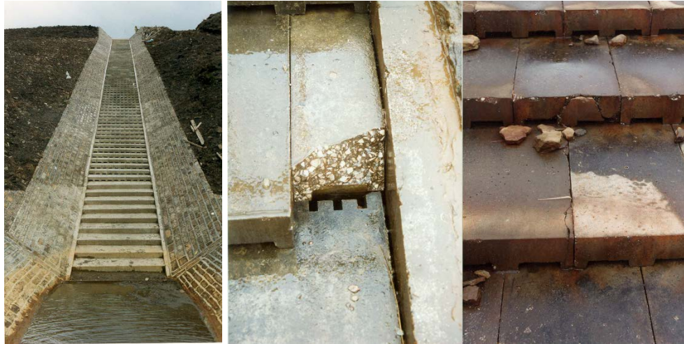
Figure 16. Brushes Clough Spillway. Left, downstream view. Center and right, WSBs with damages caused by vandalism (courtesy of R. Baker)
