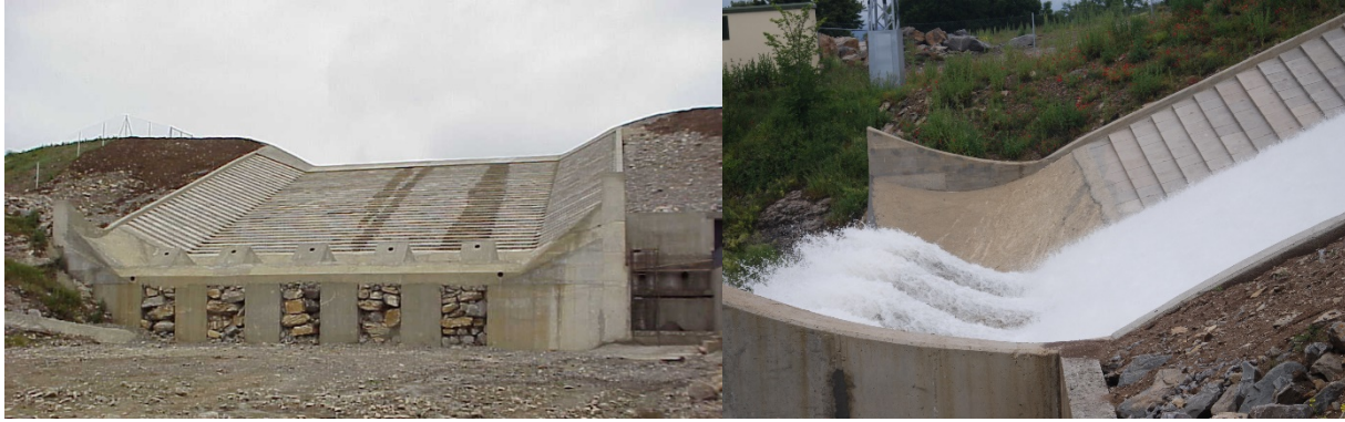
Figure 28. Flip bucket at Barriga Dam. Left, view from downstream. Right, lateral view during operation in 2008.
