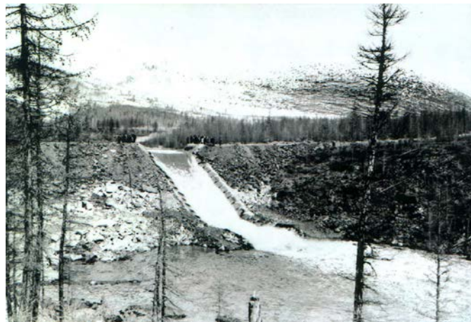
Figure 15. Picture of the spillway at embankment dam in Kolyma Project (courtesy of R. Baker)
