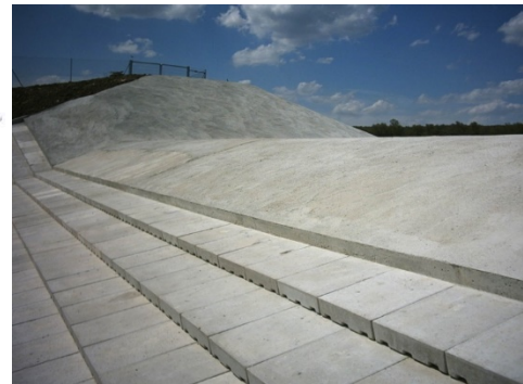
Figure 21. Crest details. Left, sketch of the cross section at Brushes Clough Dam (courtesy of R. Baker). Right, picture of downstream end of the concrete slab at the spillway crest of Barriga Dam.
