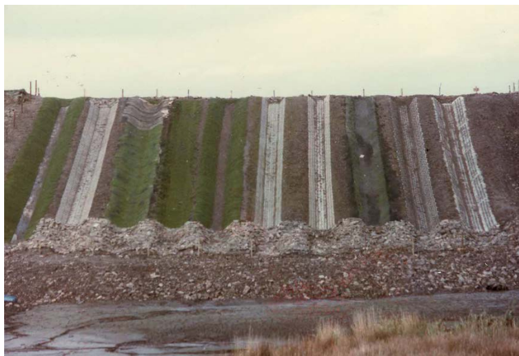
Figure 5. Experimental setup of field tests of different scour protections at Jackhouse site (Baker 1992)
