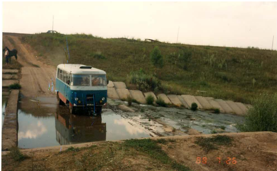
Figure 22. Bus crossing ford at the crest of Klinbeldin spillway (courtesy of R. Baker)
