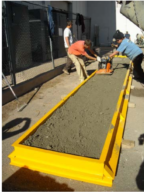
Photograph 6. Lift Compaction
