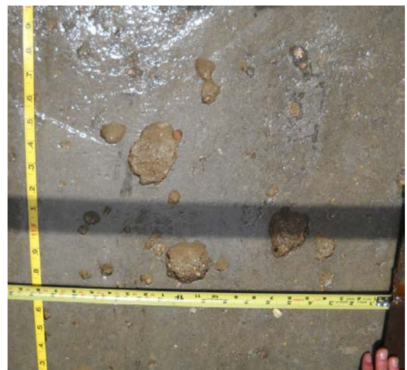
Photograph 17. Close Up – Erosion area after Test 3 – 10 Percent at 100 cfs
