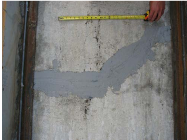
Photograph 9. Epoxy Paste Crack Repair
