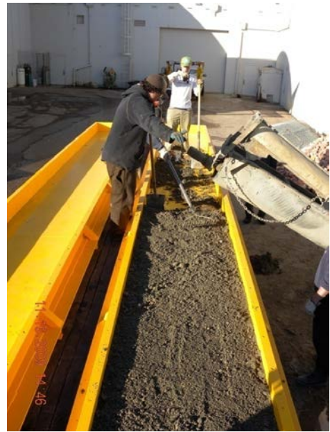
Photograph 4. First Lift Placement
