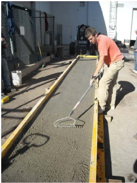
Photograph 5. Scarification between Lifts
