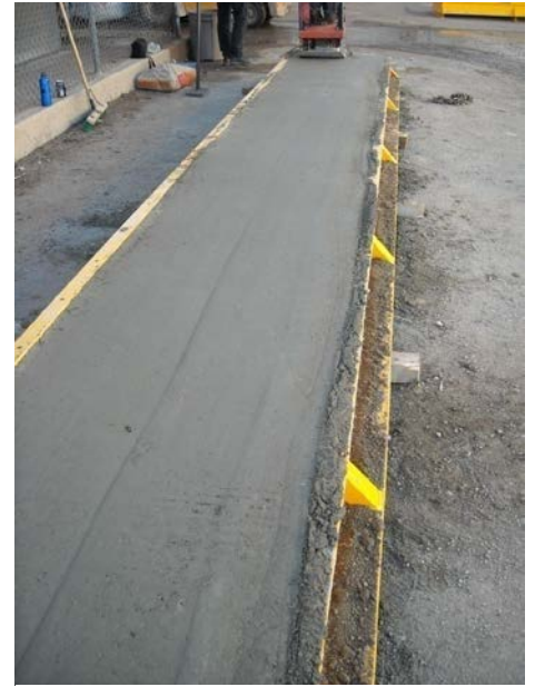
Photograph 7. Soil-cement Test Box
