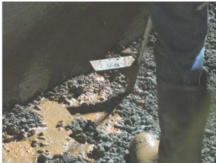
Figure 2. Method for placing grout in RCC.
