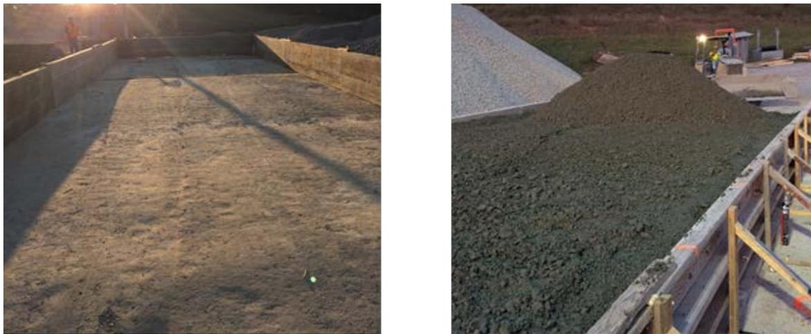
Figure 1. Formwork and construction process for GERCC field trial
