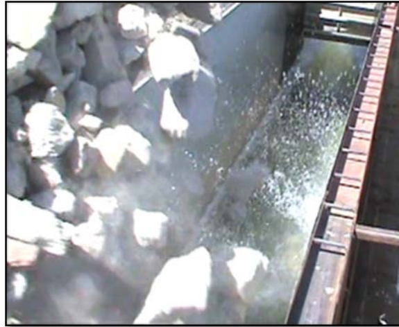
Figure 8. Broken Concrete Being Dumped into the Flume
