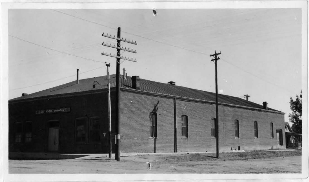
Ault School Gymnasium
