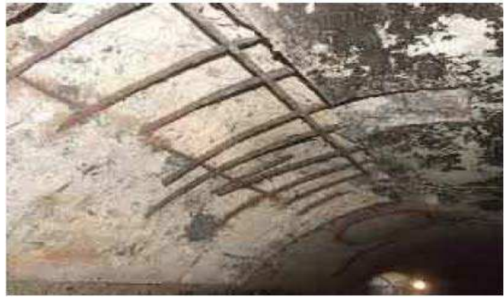
Figure 6.14: Hydrogen Sulfide Corrosion of Concrete Pipe (Dawalt)
