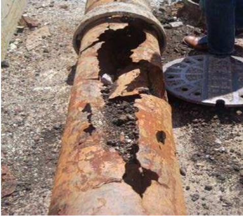
Figure 6.13: Forcemain Failure Due to H 2 S Attack (Copeland 2013b)
