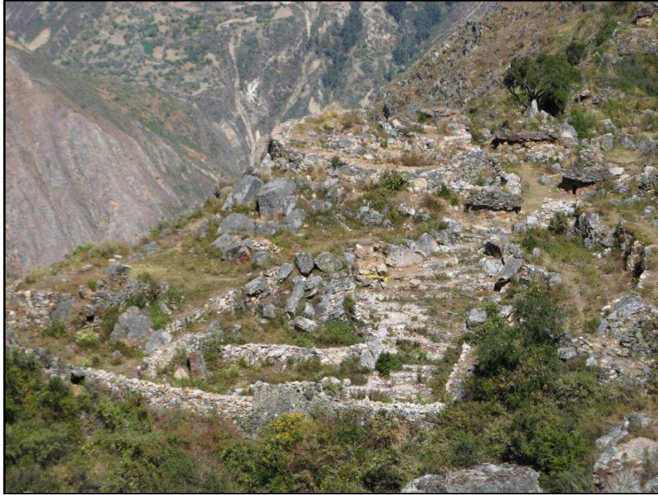
Figure 3.6. View facing south of the public sector at Marcajirca with the defensive wall, amphitheater and the tower.
