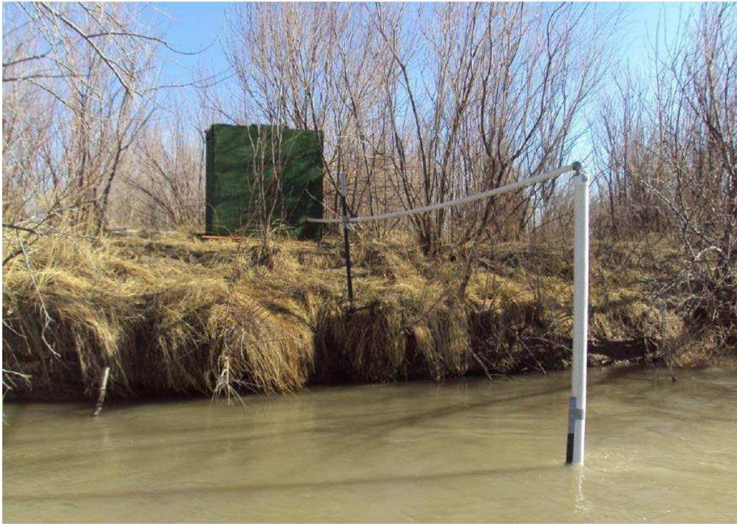
Figure 7. AquaTroll™ logger placed at the ARKD transect with cable housing structure in background (Huizenga 2015).
