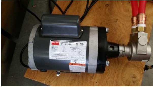
Figure 43: Circulation Pump and Motor
