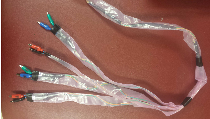
Figure 3.10. ACE1 cables in an anti-static encasing for ease of cleaning and reducing short circuit risks.
