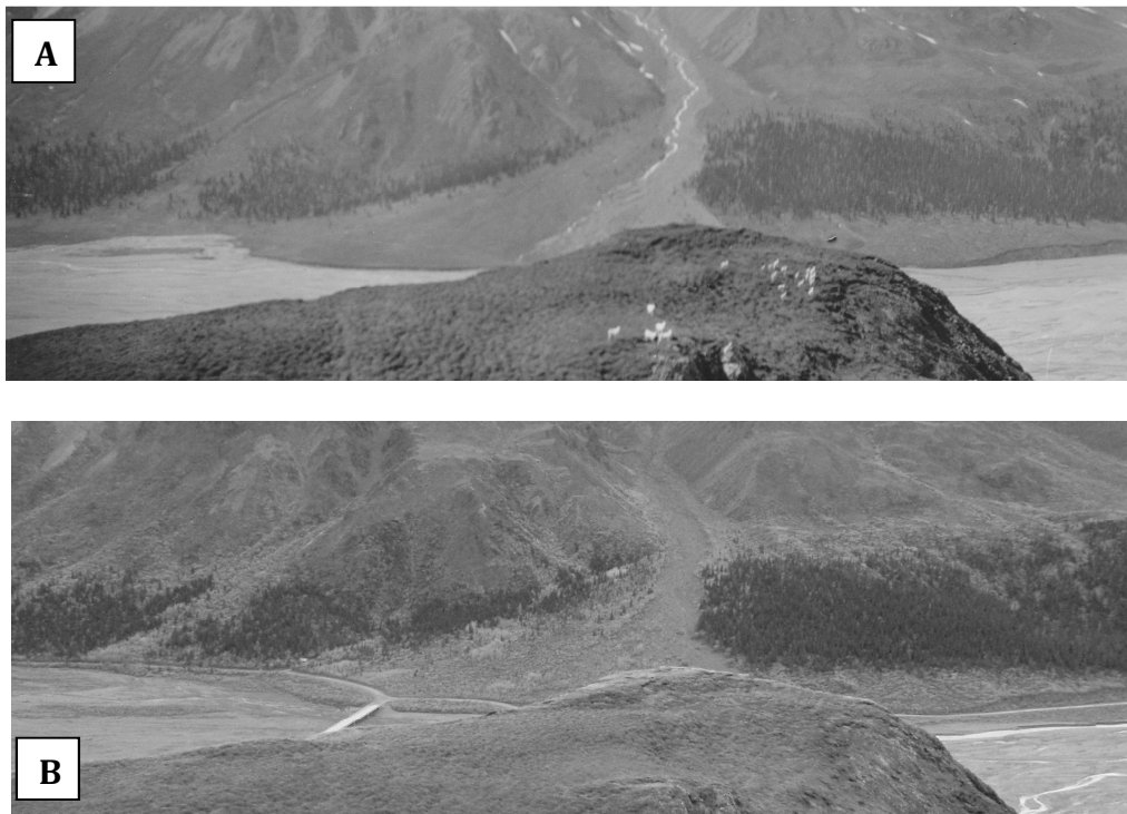
Figure 4: Image on left shows the first iteration of the East Bridge and a small section of the causeway across the Toklat River built in 1931 (NPS 1950). View is to the west and flow is left to right. Image on right shows erosion mitigation structures or revetments installed along the East Branch of the Toklat River (NPS 1982). View is to the east and flow is towards viewer. Grizzly bear for scale.
