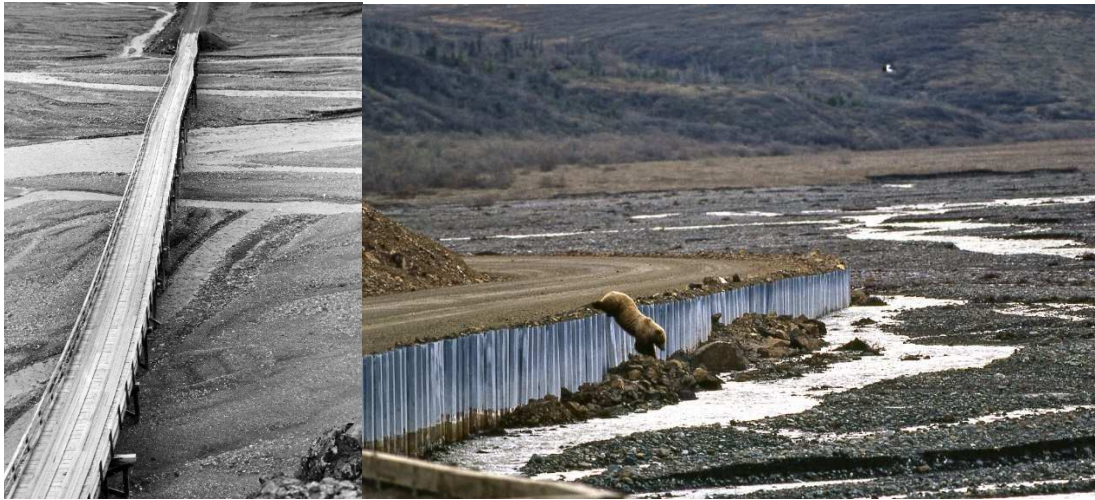
Figure 4: Image on left shows the first iteration of the East Bridge and a small section of the causeway across the Toklat River built in 1931 (NPS 1950). View is to the west and flow is left to right. Image on right shows erosion mitigation structures or revetments installed along the East Branch of the Toklat River (NPS 1982). View is to the east and flow is towards viewer. Grizzly bear for scale.
