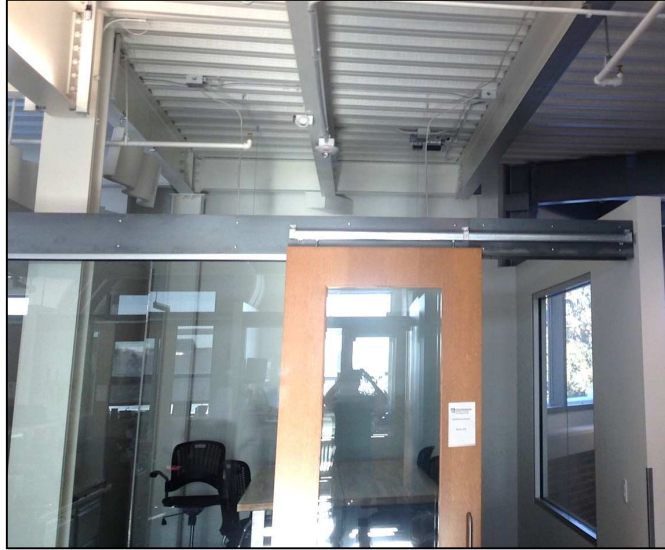
Figure 6.2: Example of the open-ceiling office design shared by all offices on the second and third floors.
