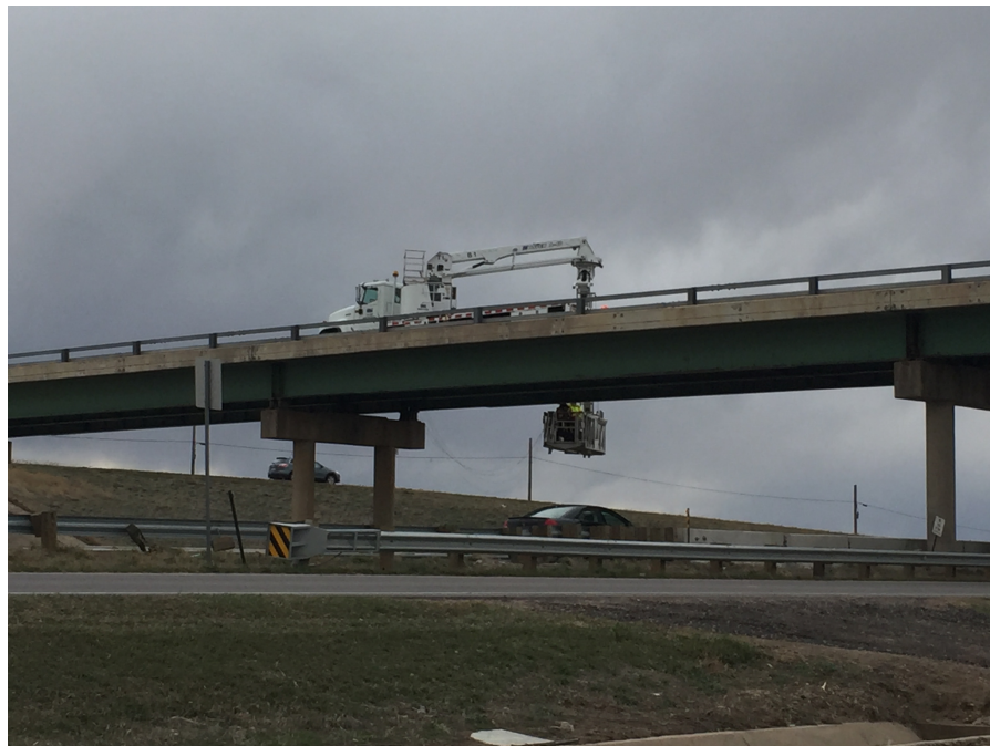
Figure 3-9. Aspen Aerial A-40 Snooper Truck on B-16-FM
