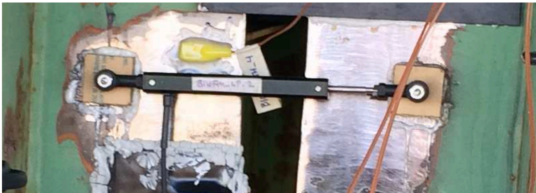
Figure 3-17. Installed thermocouple on B-16-FM to Measure Relative Displacement between Girder Ends
