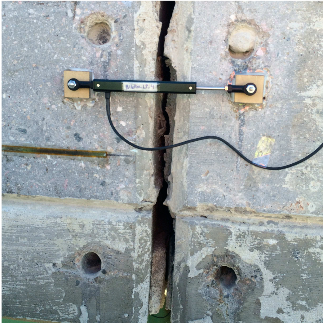
Figure 3-13. Linear Potentiometer Installed to Measure Relative Displacement at Deck Level
