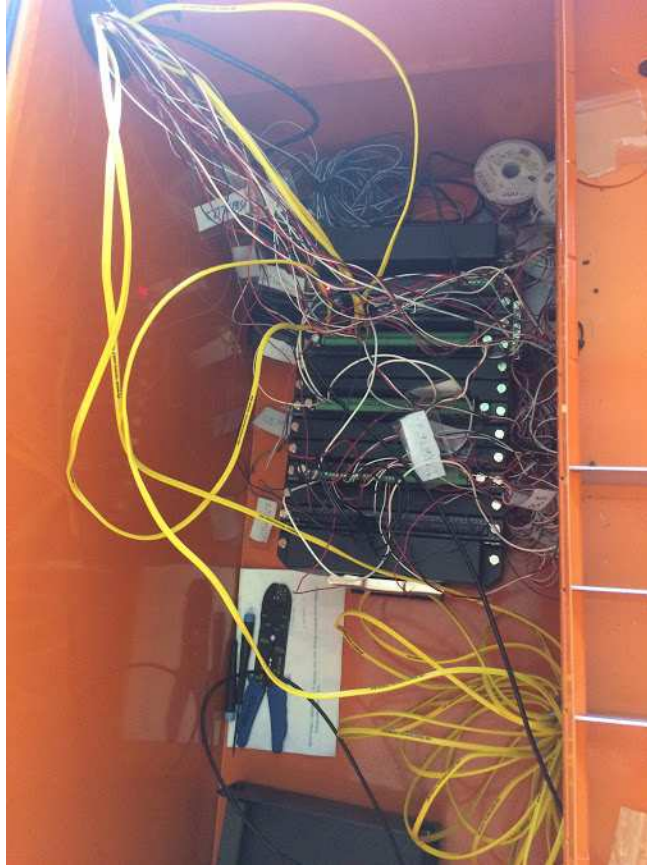
Figure 3-23. Inside of Weather Tight Job Box Containing CR9000X Data Logger
