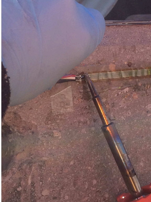
Figure 3-19. Soldering Quarter Bridge wires to Concrete Strain Gauge
