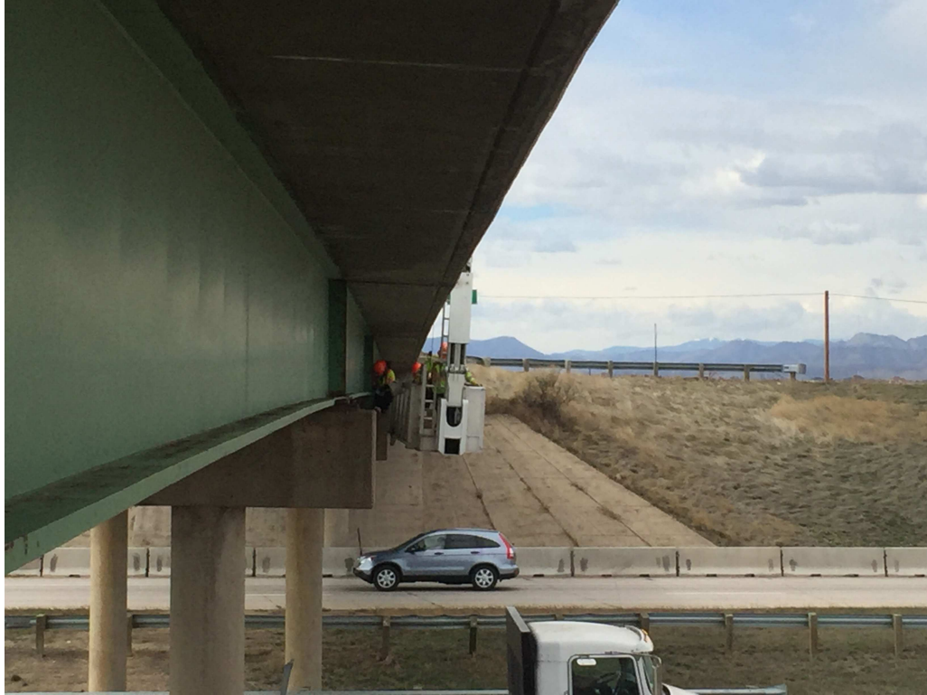
Figure 3-10. Snooper Truck in Position for Instrumentation
