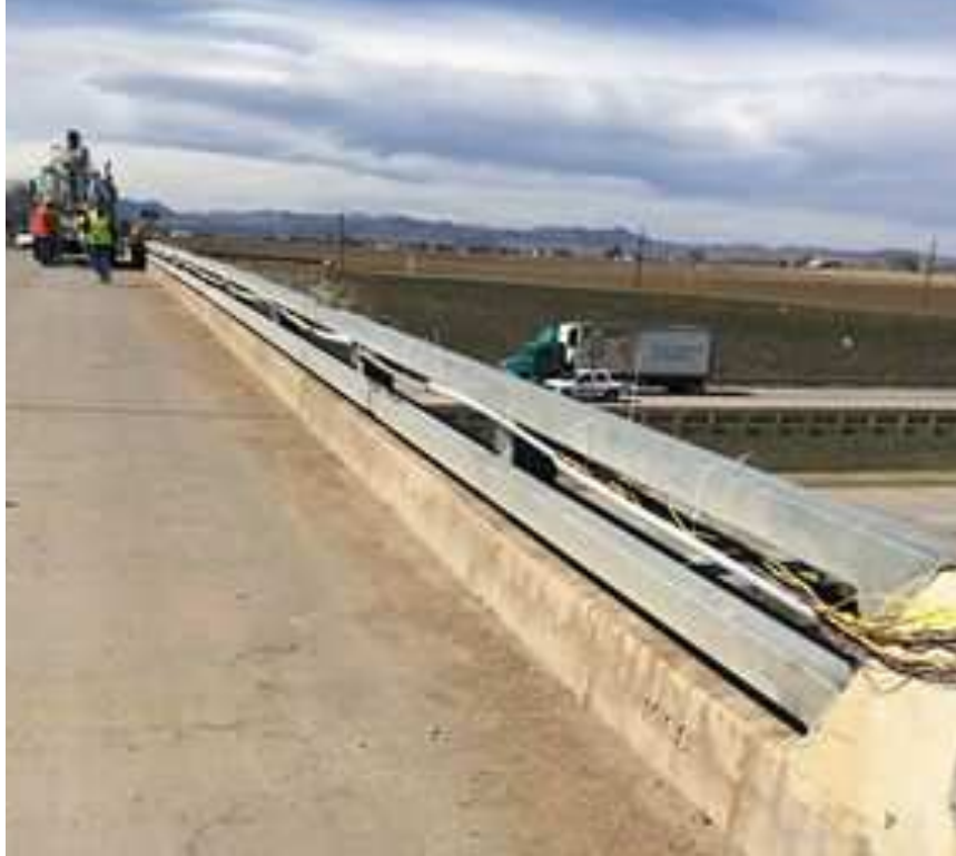
Figure 3-24. Wires Placed in PVC pipe and Secured to the Guard Rail
