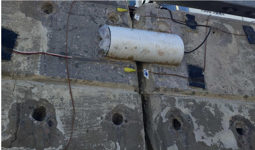
Figure 3-14. Linear Potentiometer covered by PVC pipe
