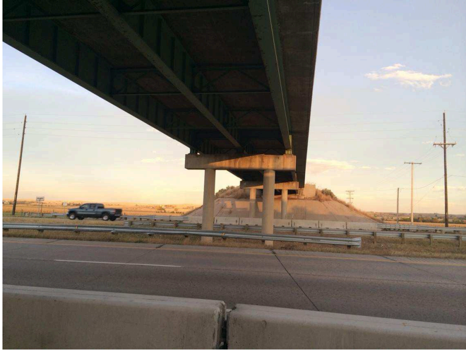
Figure 3-2. B-16-FM Superstructure from the West Abutment (photo by Author)
