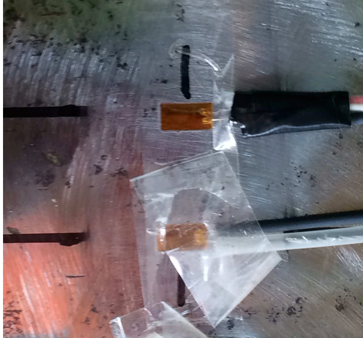
Figure 3-20. Initial Installation of Strain Gauges on Bottom Flange on B-16-FM
