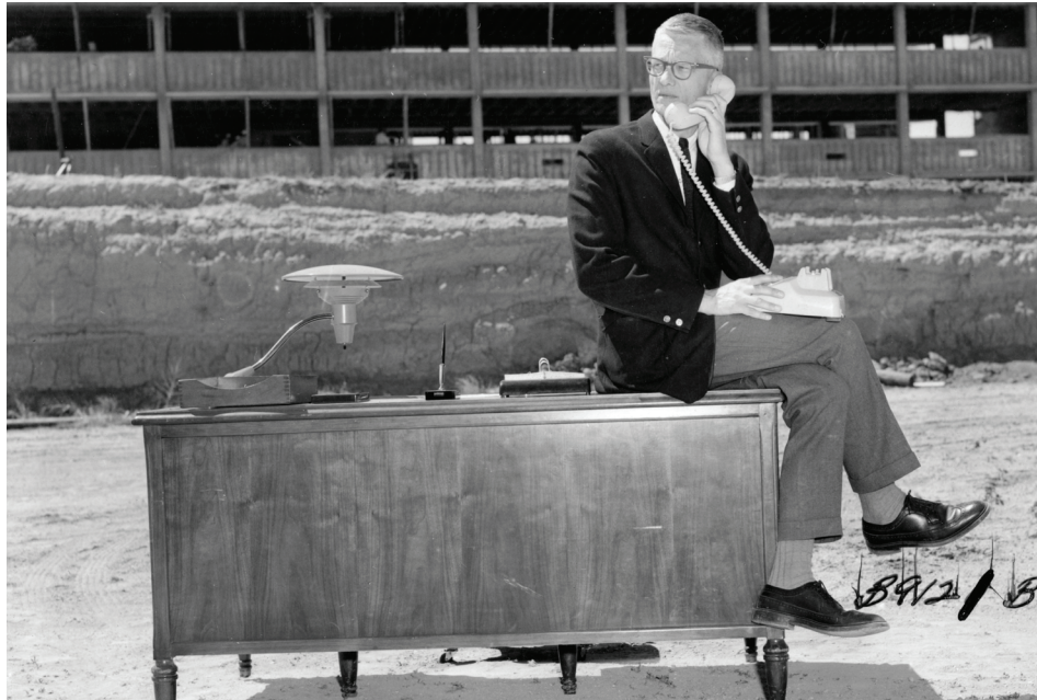
Lee Anderson 'working' at his desk at the Morgan Library construction site, c. 1964
