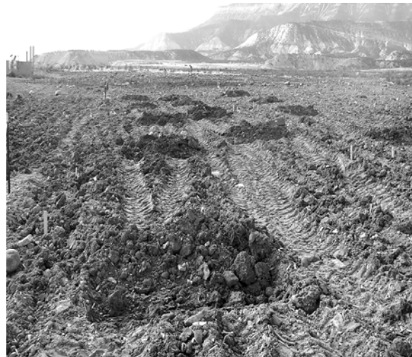
Fig 1. Finished micro-catchments on rough seedbed treatment on reclamation test plots on the Western Slope of Colorado.
