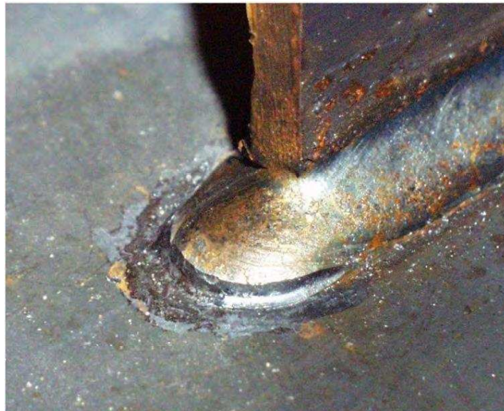
Figure 10. Air hammer peening for repairing fatigue cracks; after: Dexter (2005)
