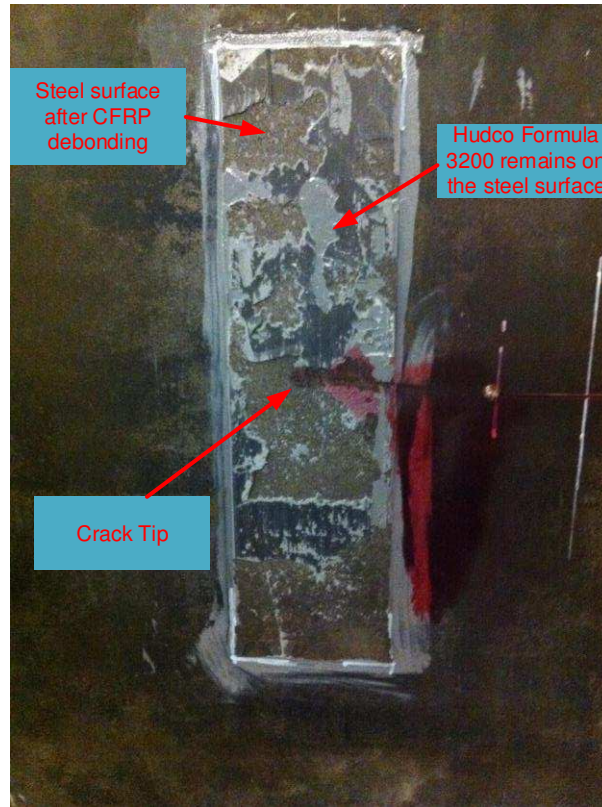
Figure 45. Steel surface after CFRP debonding (front left) at 378,756 cycles for specimen 2
