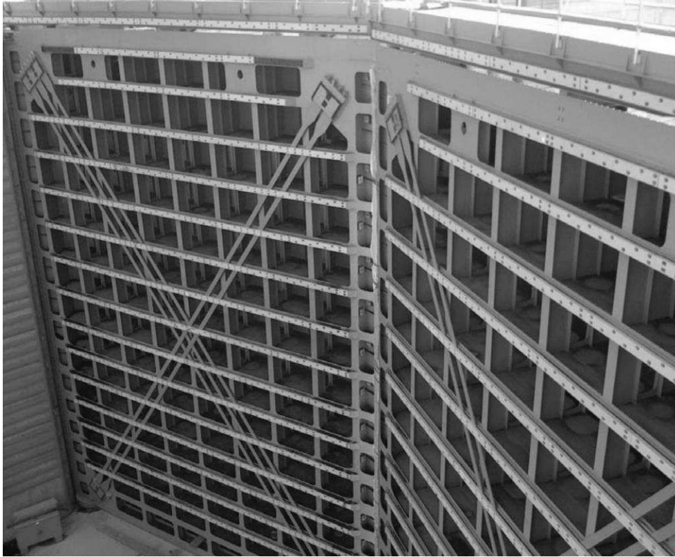
Figure 1. Typical horizontally framed miter gate; source: HQUSACE (2010)
