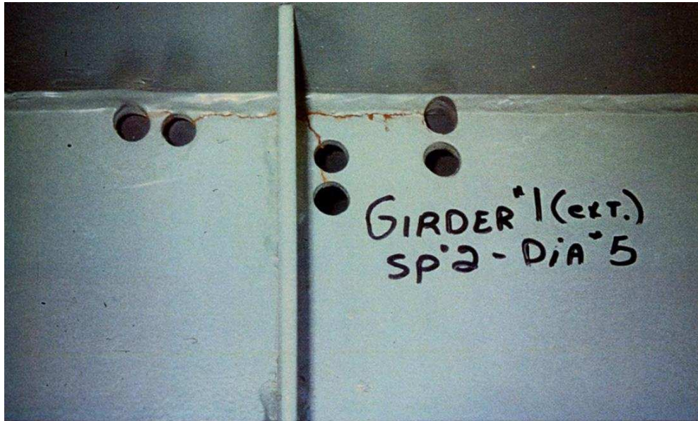
Figure 11. Hole drilling method to stop crack propagation; after: Dexter (2005)
