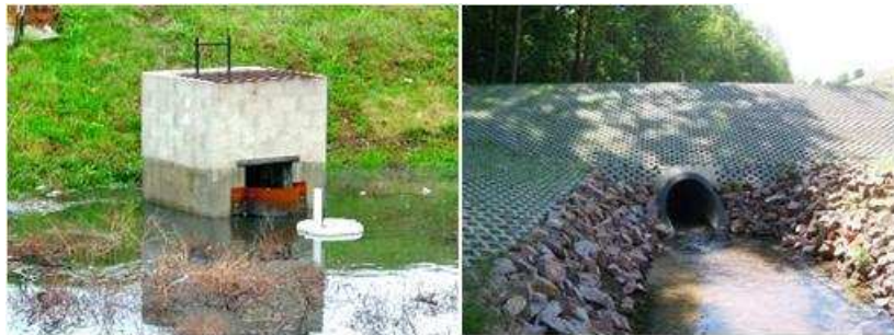
Figure 10: Examples of a) extended detention basin and b) flood control basin
