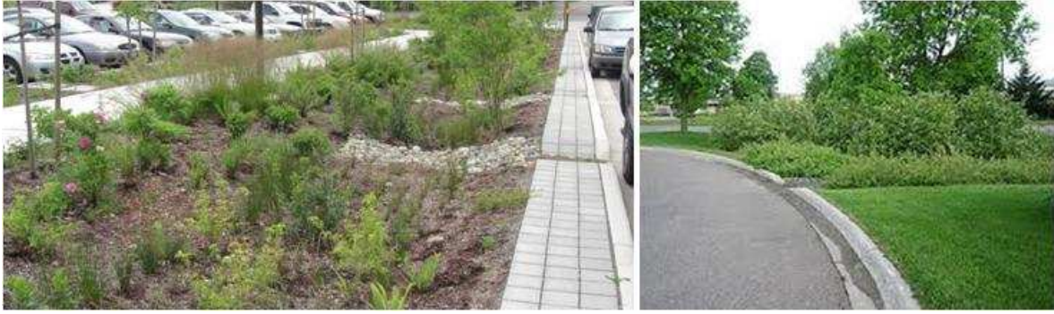
Figure 9: Examples of Bioretention Basins along a) a parking lot median and b) a roadside parkway
