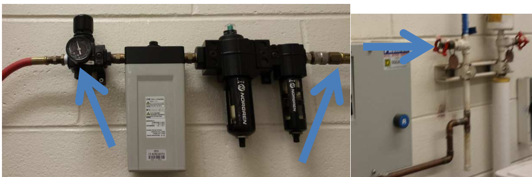
Figure 6.10: Pressure source, regulator, and connection.
