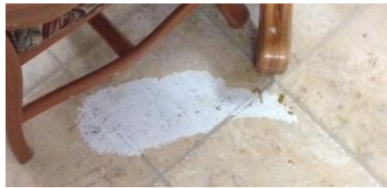
Figure 13. Significant wear of flooring in kitchen/activity area.
