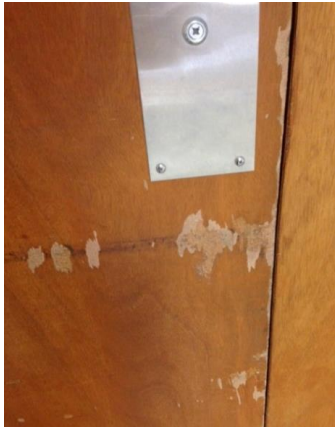
Figure 15. Door surface wear.
