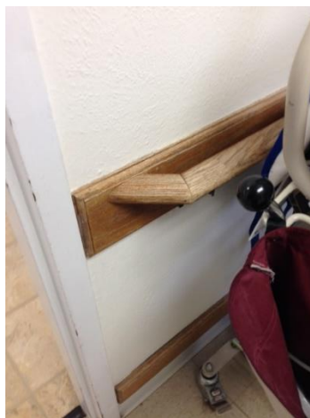
Figure 14. Chipped frame of opening.
