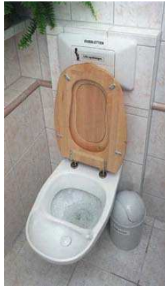
Figure 7 Dubbletten urine diversion toilet
