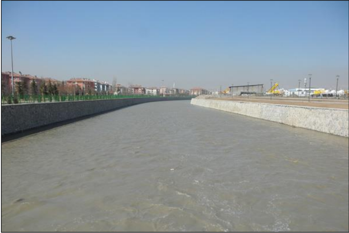
Figure 7: Stabilized portion of Ankara River along the town of Ayas
