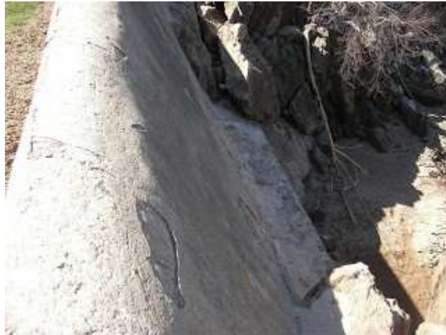
Figure 5.6 Abandoned dam, Baja California Sur, April 2013. Source: Haeffner, 2013.
