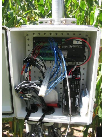
Figure A.5: Photograph of weatherproof box containing data loggers connected to sensors.
