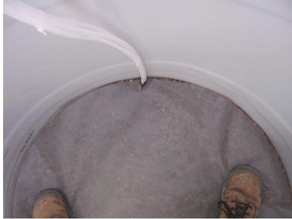
Figure A.11: Photograph of metal screen and weed-blocking fabric placed on top of the pea gravel reservoir in the lysimeters.
