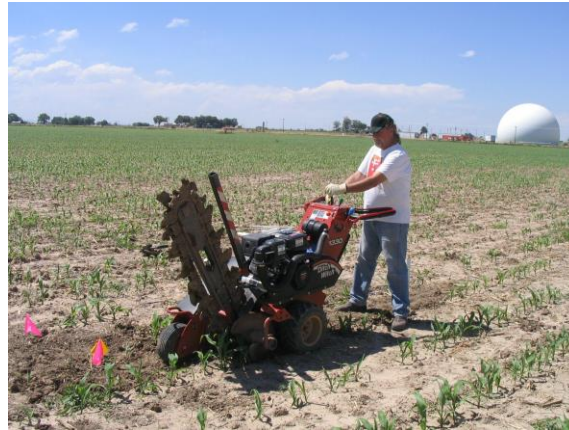
Figure A.4: Photograph of equipment used to create trench for burying wires and guiding the wires to the stickup pipe in the adjacent row.
