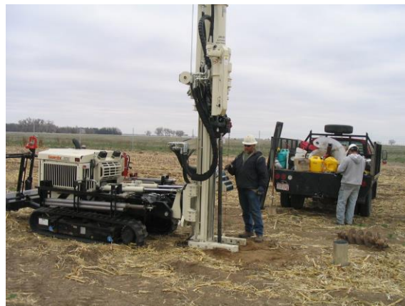
Figure A.13: Photograph of the push-point drill used to install the combination water table monitoring wells and neutron probe access tubes.
